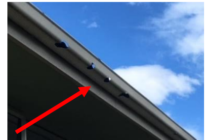
Hail damaged PVC gutter
